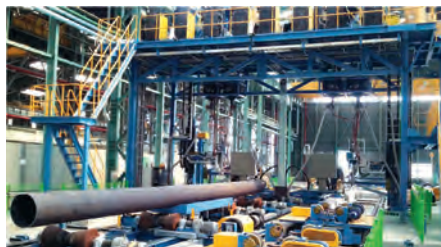
Outside Welding Machine
